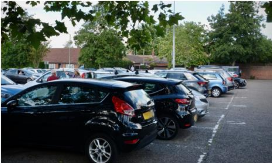
Good delineation of different areas will assist motorists. This is Long Stay – but not clearly defined as the legend is illegible at this size, and has worn away
